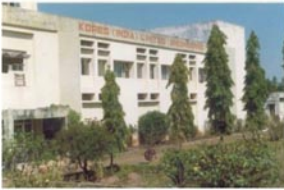
KORES INDIA LTD manufacturing facility at Pithampur, INDIA
